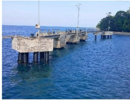
Gambar II.18 Breasthing dan Mooring Dolphin
