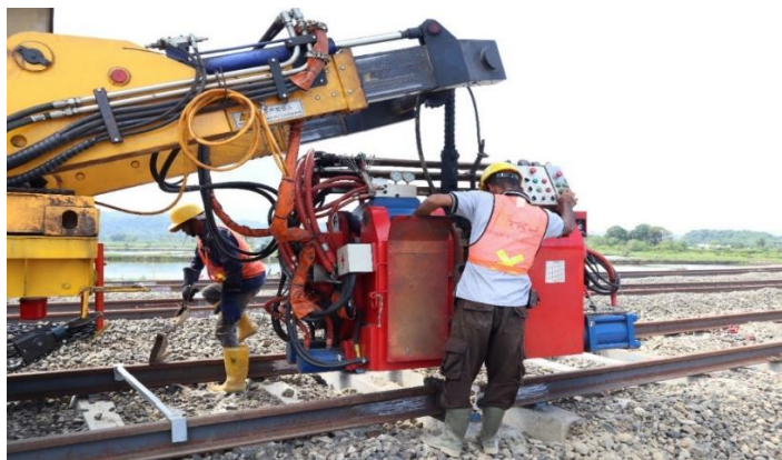
Gambar III. 5 Proses Pengelasan Flashbutt
