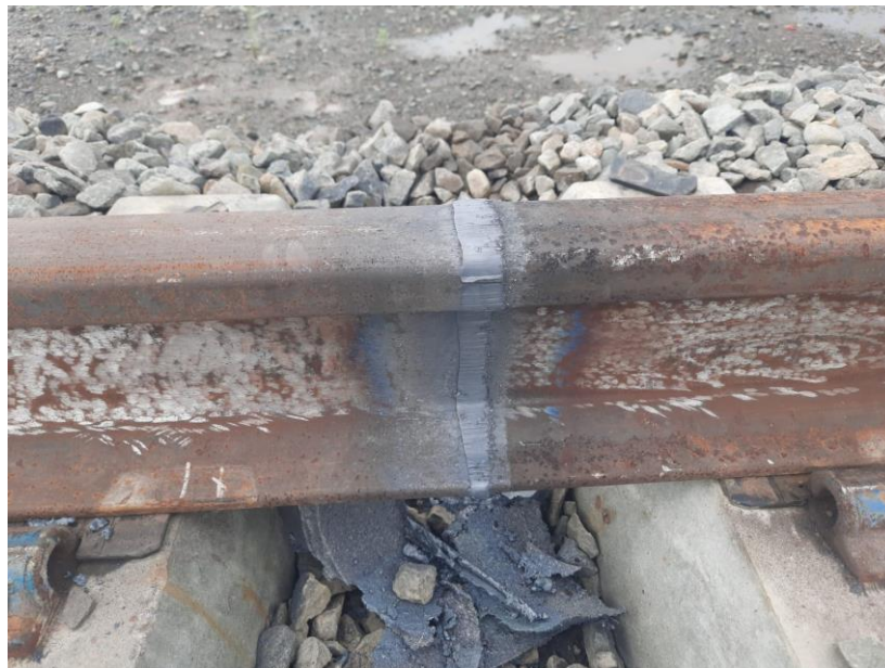
Gambar V. 1 Hasil Pengelasan Metode Flashbutt
