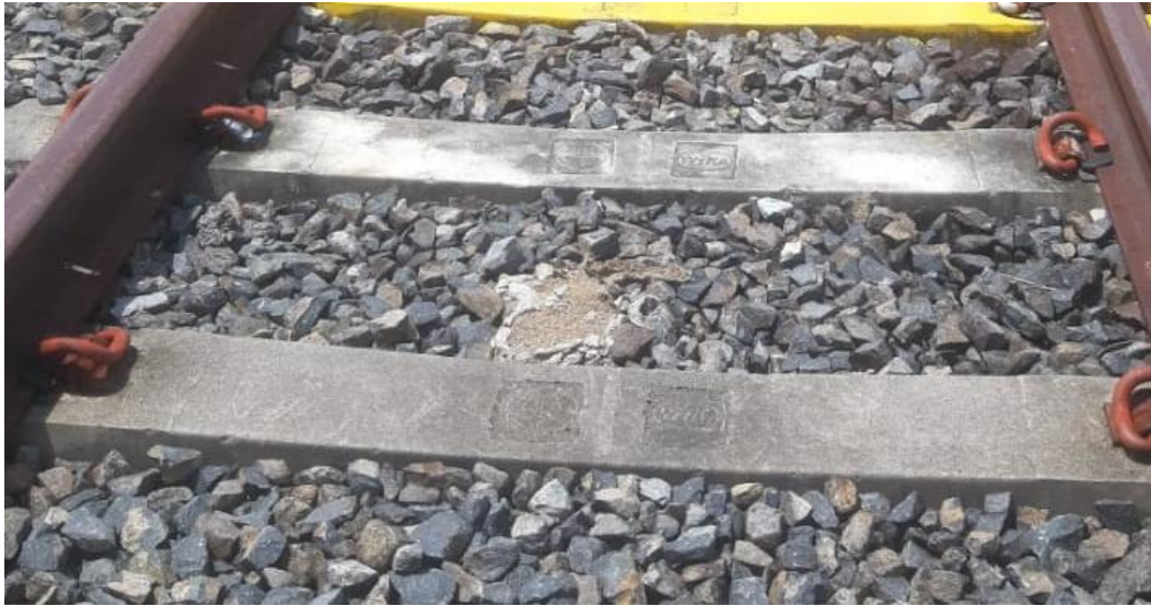
Gambar II. 4 Bantalan Beton
