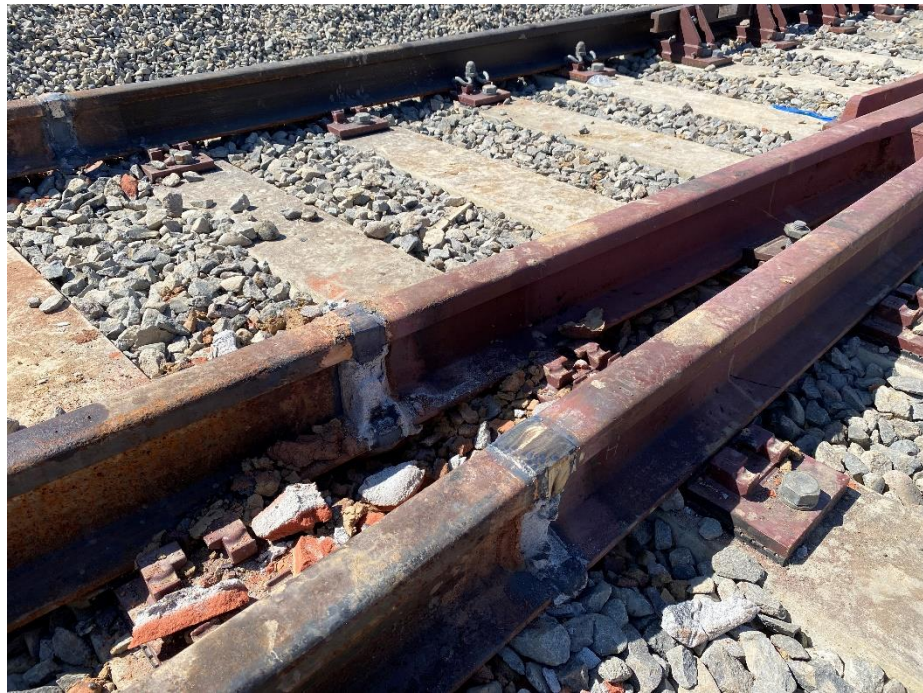
Gambar V. 2 Hasil Pengelasan Metode Thermit
