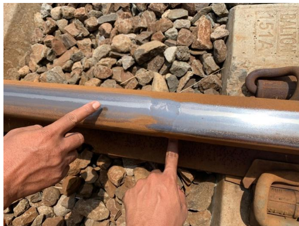
Gambar V. 1 Rel defect KM 26 + 451
