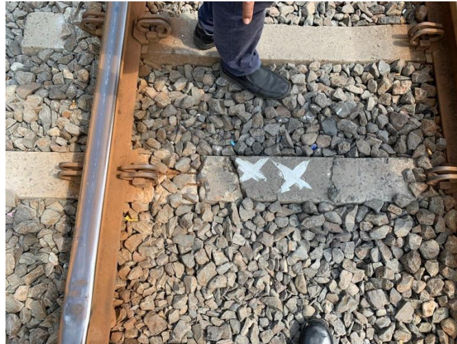
Gambar V. 3 Bantalan Retak Prioritas II KM 25 + 310
