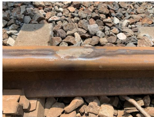
Gambar II. 5 Rel Defect KM 26 + 317
