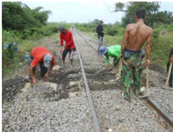
Gambar V. 12 Gambar Kuras Mud Pumping
