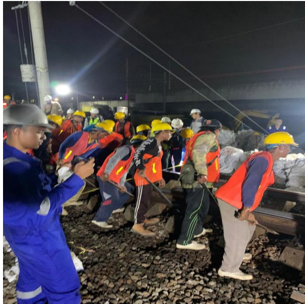
Gambar V. 7 Proses shifting jalur eksisting ke jalur permanent
