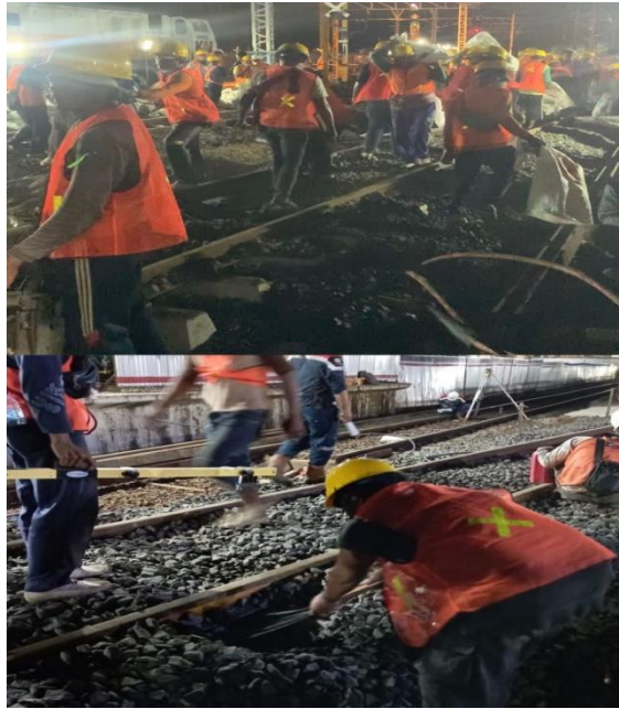
Gambar V. 10 Proses pengisian dan perataan ballast
