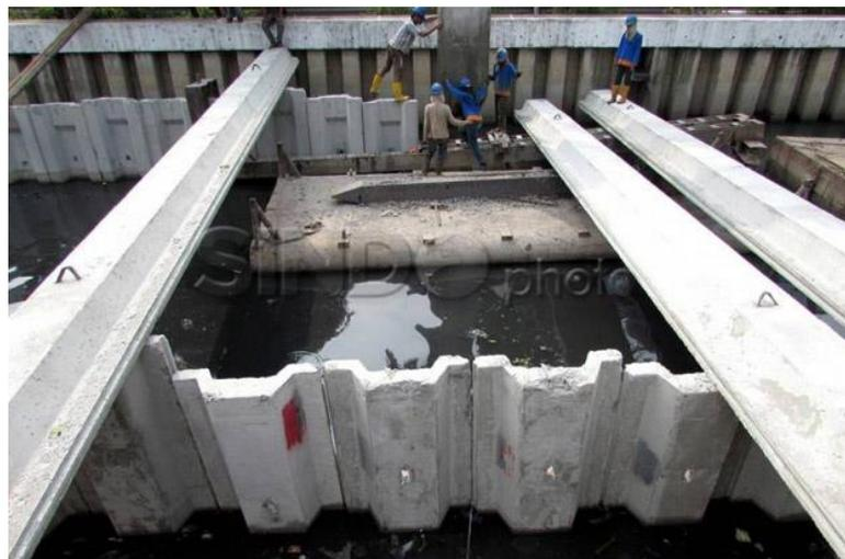
**Gambar III. 5** *Sheet pile* beton
