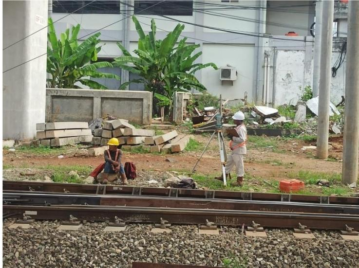
**Gambar V. 4** *Stacking Out*
