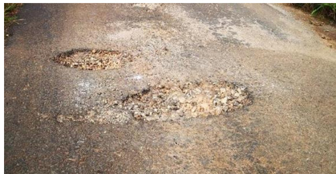
Gambar III.4 Lubang ( Photoles )
