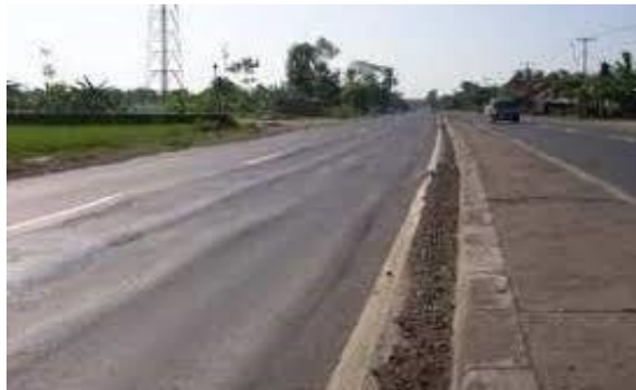
Gambar III.8 Alur/Rutting
