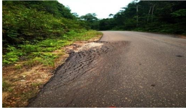
Gambar III.5 Cacat Tepi Perkerasan
