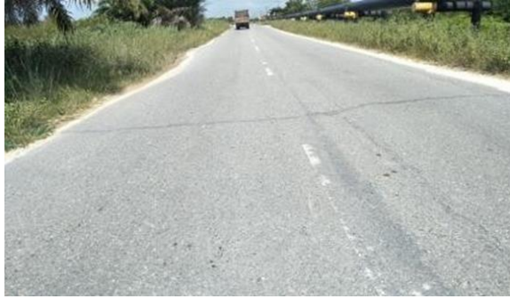
Gambar III.7 Retak Melintang
