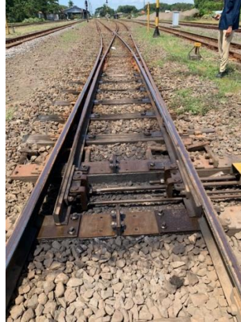
Gambar II. 12 Rel Lantak
