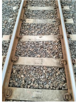
Gambar II. 3 Bantalan Beton
