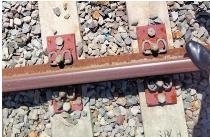
Gambar II. 6 Penambat Fast-Clip KM29 +721
