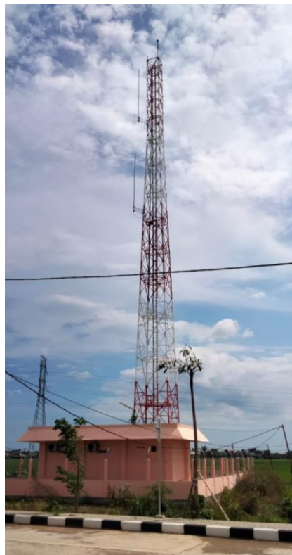
Gambar V. 8 Radio Base Station Rammang-rammang
