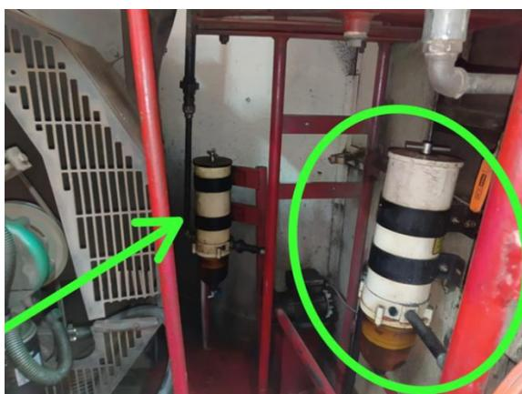
**Gambar 2** Kondisi Genset 2 *Filter racor*
