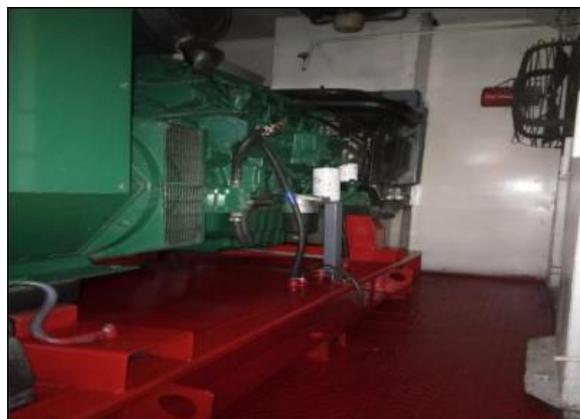
**Gambar 3** Kondisi Genset Tanpa *Filter racor*
