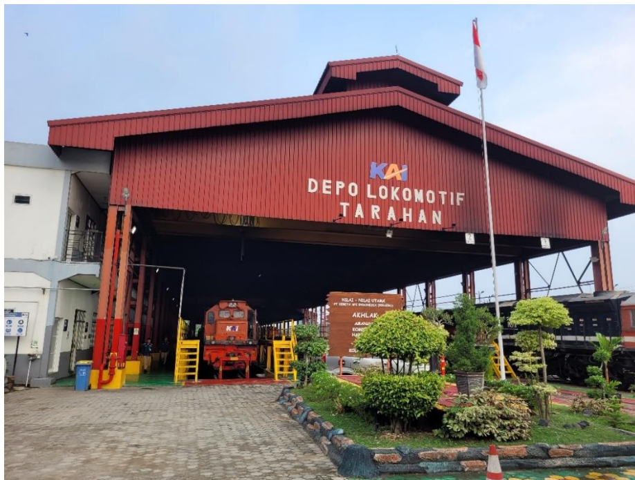
Gambar II. 4 Depo Lokomotif Tarahan
