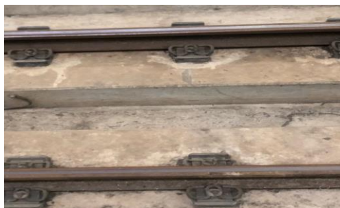
Gambar II. 7 Bantalan Slabtrack
