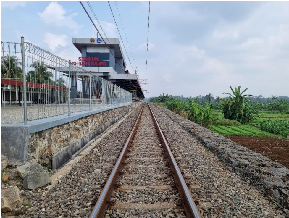
Gambar II. 6 Jalan Rel Km 41+500 Lintas Citayam–Nambo
