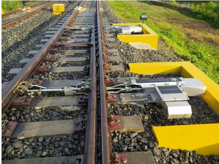
**Gambar II. 14** *Point Machine* Voestalphine UNISTART HR EM
