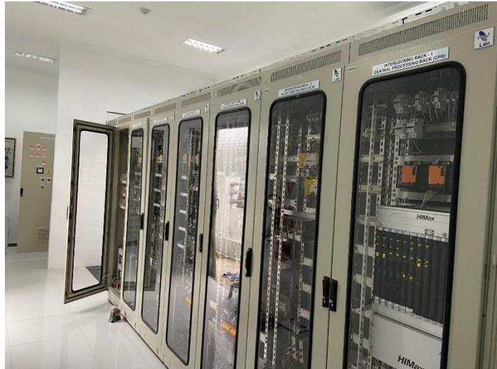
**Gambar II.6** *Interlocking* SiLSafe 4000
