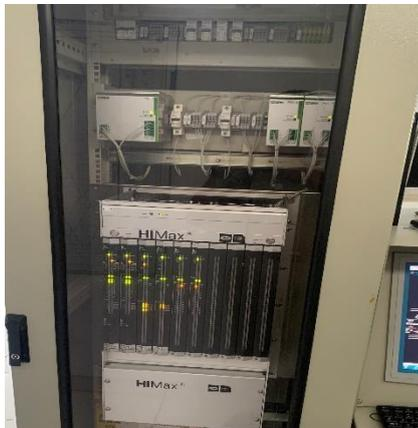
**Gambar II. 7.** *Programmable Logic Controller (PLC)*
