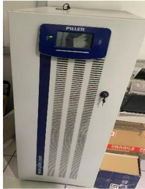
**Gambar II. 11.** *Uninterruptible Power Supply (UPS)*
