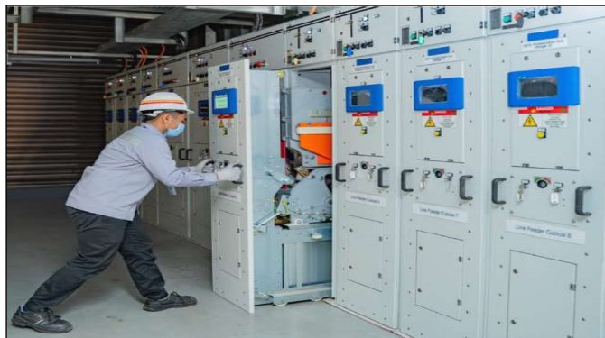
Gambar II. 15 Peralatan DC Switchgear
