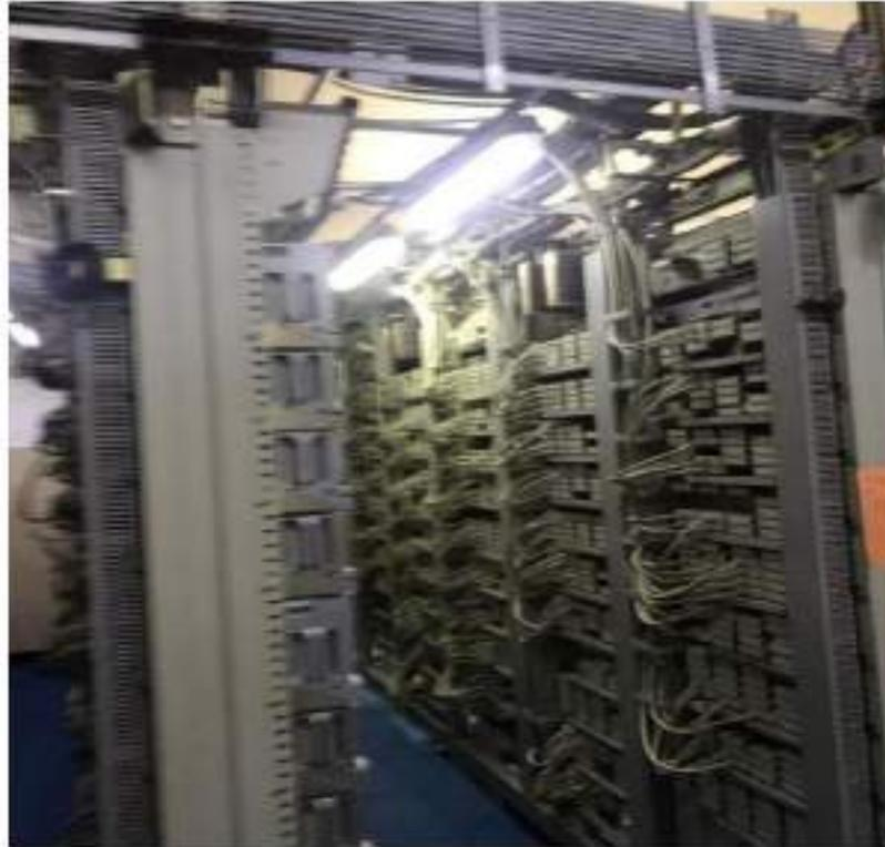
**Gambar V. 1** Rak Interlocking MIS 801
