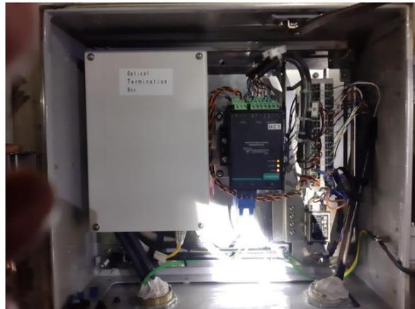
**Gambar II.10** *Station Computer Interface (SC – IF)*
